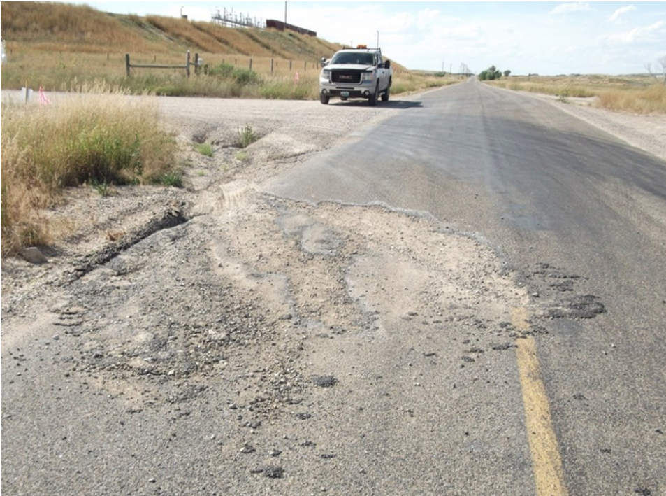
Damage to Road that had been chip sealed over gravel. It appears that a low boy made a short turn and bottomed out, scraping away the road surface.
