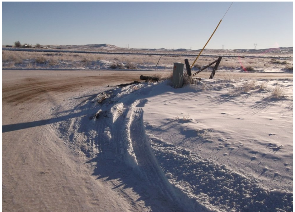
Sign run over, oil tankers come to this intersection and have to turn right. Damaged a couple of times.
